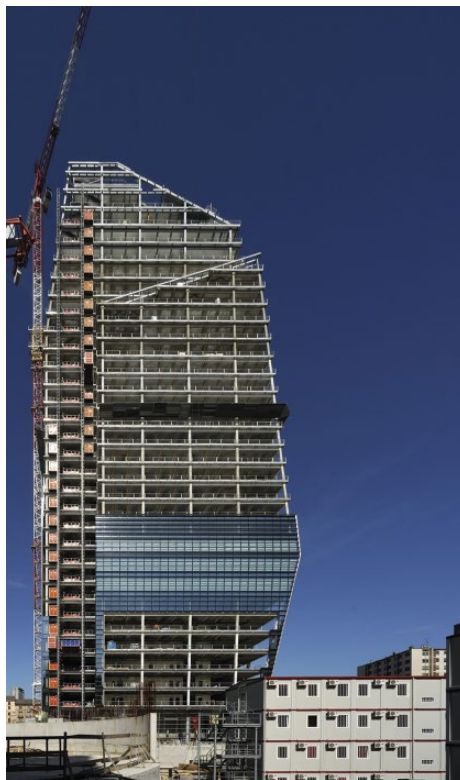
Figure 3 Construction phase – the steel structure is already finished. © Oskar Da Riz / Stahlbau Pichler.
