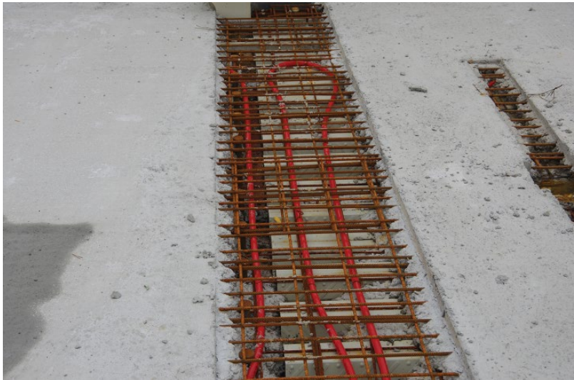
Figure 4.83 Composite floor with embedded pipes.
