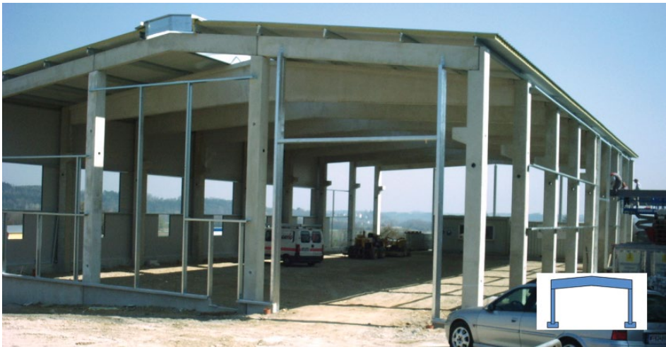
Figure 6.6 Single-storey building with a precast RC frame, symbol for RC frame. © Dr. Gerhard Köhler, Werksvertretungen.
