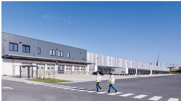
Figure 1 Sandwich facade on the DSV logistics building in Krefeld, Germany. © Goldbeck.
