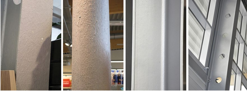
Figure 4.55 Where no or only minor requirements are made on the visual appearance of a fire-protective coating, the most suitable finish standards are Q1 (left). Decorative finishes (Q3) meet highest demands on their surfaces (right). © AkzoNobel.
