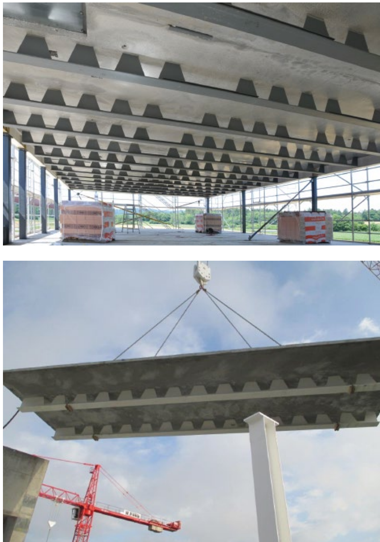
Figure 4.19 Spanning a building without columns using a TOPfloor INTEGRAL composite deck – view of underside of deck and installation of element. © H. Wetter AG, CH-Stetten.
