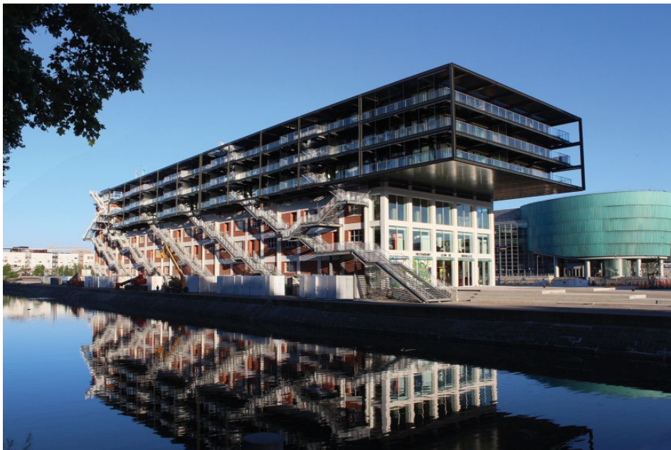
Figure 1 On the northern facade, fire escapes are externalized, connecting the different uses with some structural acrobatics. © Heintz-Kehr Architectes.
