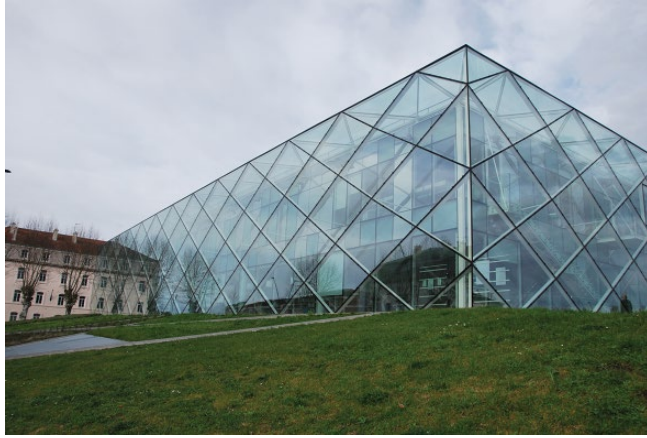
The reflecting and transparent façade. © ConstruirAcier.
