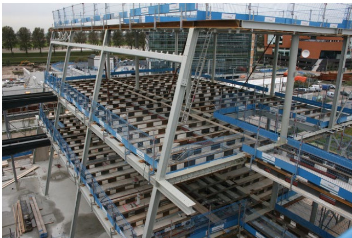
Figure 2 During the construction phase – the hole pattern in the steel beams of the Slimline floor system for accommodation of all common building installations is still visible. © Slimline Buildings.
