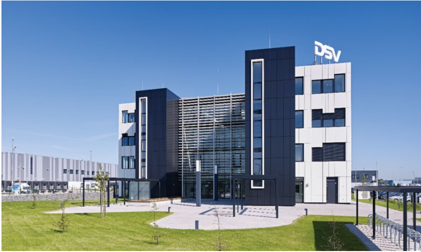
Figure 2 Aluminium cassette façade. © Goldbeck.
