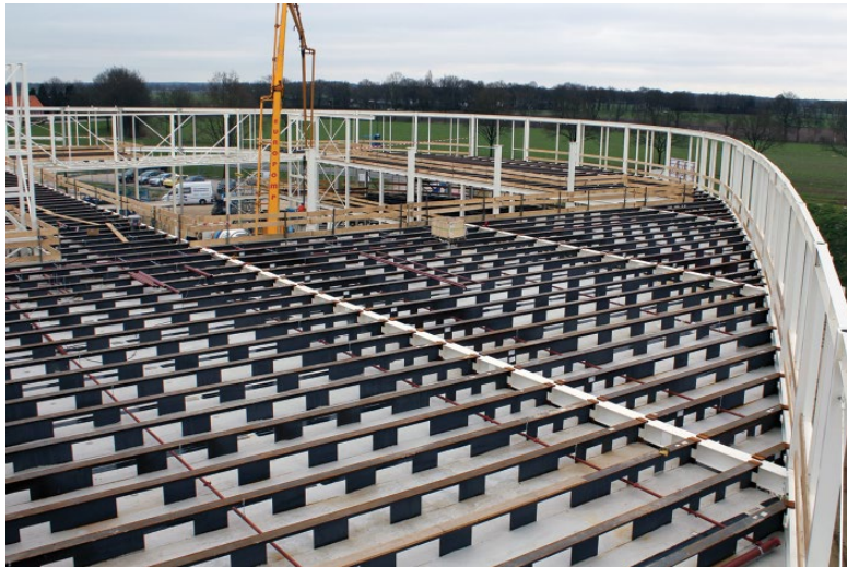
Figure 2 Slimline floor elements with steel beams allow special building shapes, like the egg-shaped Venco Campus. © Slimline Buildings.
