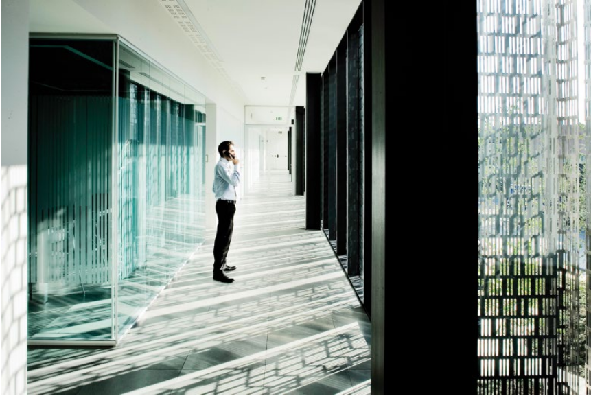
Figure 2 The stainless steel facade provides natural lighting. © Filippo Romano/Stahlbau Pichler.
