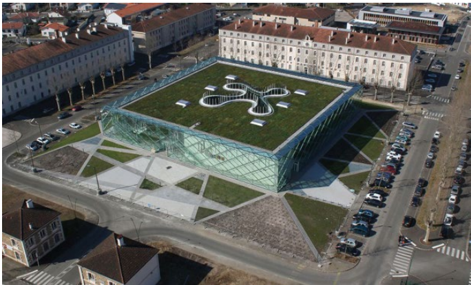
Figure 1 Aerial view of the building. © Marsan Agglomeration.
