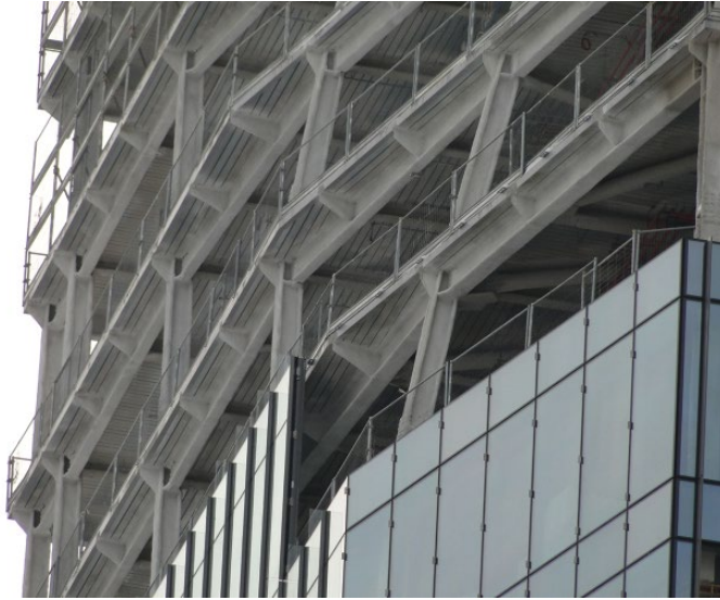
Figure 2 Steel structure with inclined columns. © bauforumstahl.
