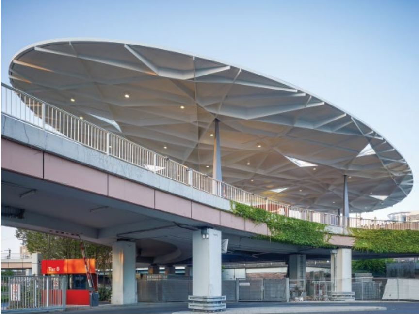
Figure 3.12 Oval roof of the north entrance to the Frankfurt trade fair grounds, Architecture: Ingo Schrader Architekt BDA, Structural Design, Physics and Sustainability: Bollinger + Grohmann. Photo: © Christian Richters.
