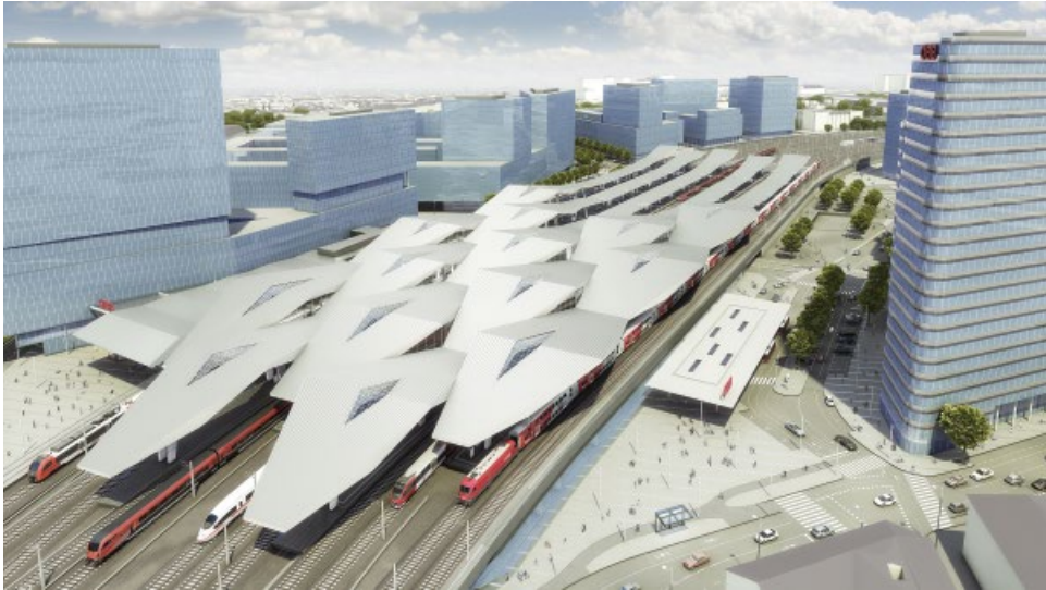
Figure 3.8 Integrated planning played a central role in the construction of the new roof of the Vienna railway station with its diamond-shaped trusses (simulation). © ÖBB/Stadt Wien.
