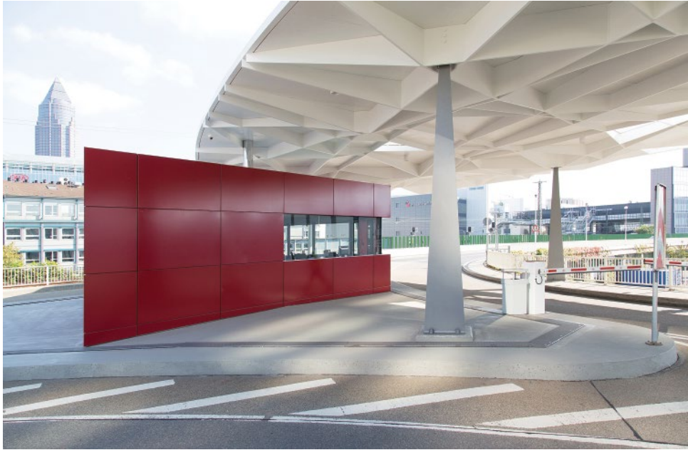
Figure 3.14 Oval roof of the north entrance of the Frankfurt trade fair grounds, Architecture: Ingo Schrader Architekt BDA, Structural Design, Physics and Sustainability: Bollinger + Grohmann. © Ingo Schrader Architekt BDA.
