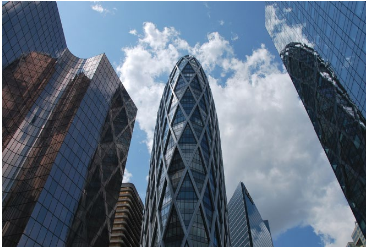
Figure 3 External diagrid structure with its diamond-shaped windows creates a unique lighting effect. © ConstruirAcier.
