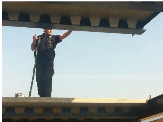
Figure 4 Construction phase – rapid construction with prefabricated TOPfloor INTEGRAL elements. © H. Wetter AG.
