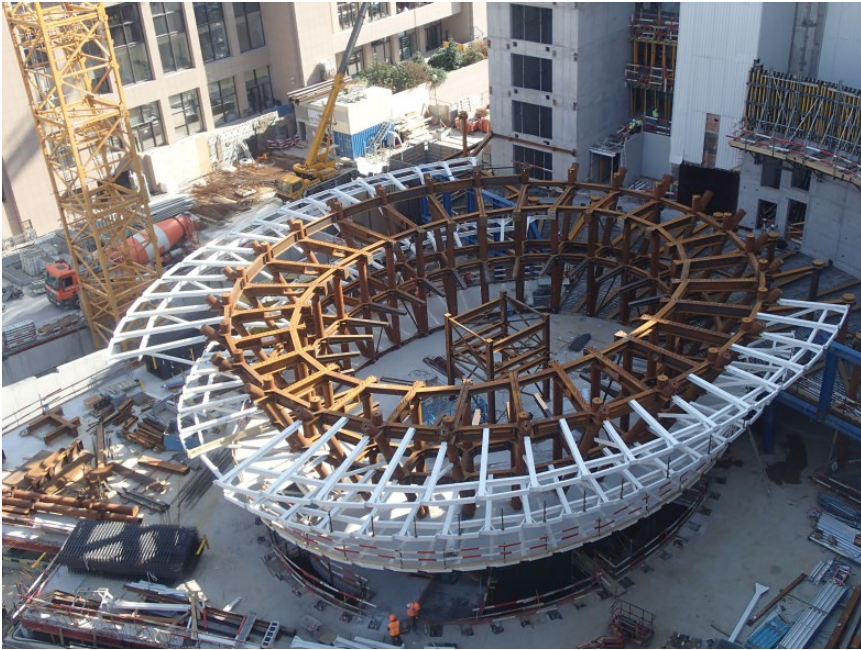
Figure 2 Growing steel structure of the inner lantern-shaped volume. © Thierry Henrard.
