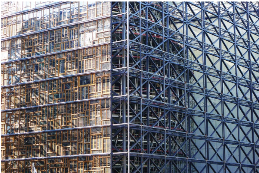
Figure 3 The new double facade, made of a harmonised patchwork of reused old oak windows, provides the necessary acoustic barrier from the traffic noise and offers a first thermal insulation for the inner space. © Thierry Henrard.
