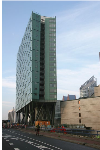
Figure 1 La Fenêtre, The Hague. © Slimline Buildings.
