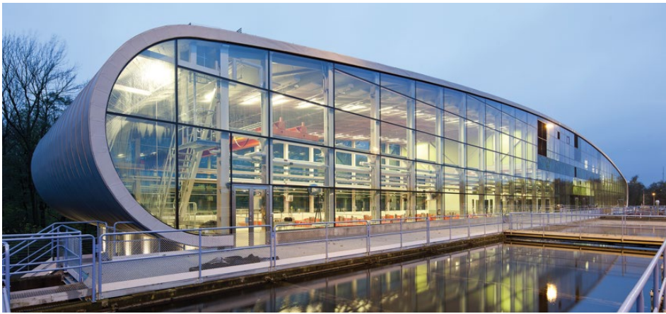
Figure 1 Rya Wastewater Treatment Plant. © Kasper Dudzik.
