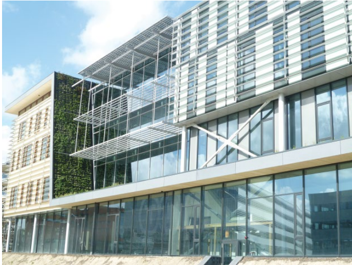
Figure 1 Bosch Siemens Experience Center, Hoofddorp. © Slimline Buildings.
