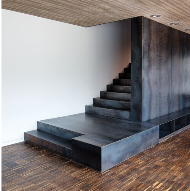
Figure 4.6 ‘Metallwerkstück’ (metal workpiece). Architects: m.schneider a.hillebrandt office building Bad Laasphe, Germany, 2010 © Cornelis Gollhardt.
