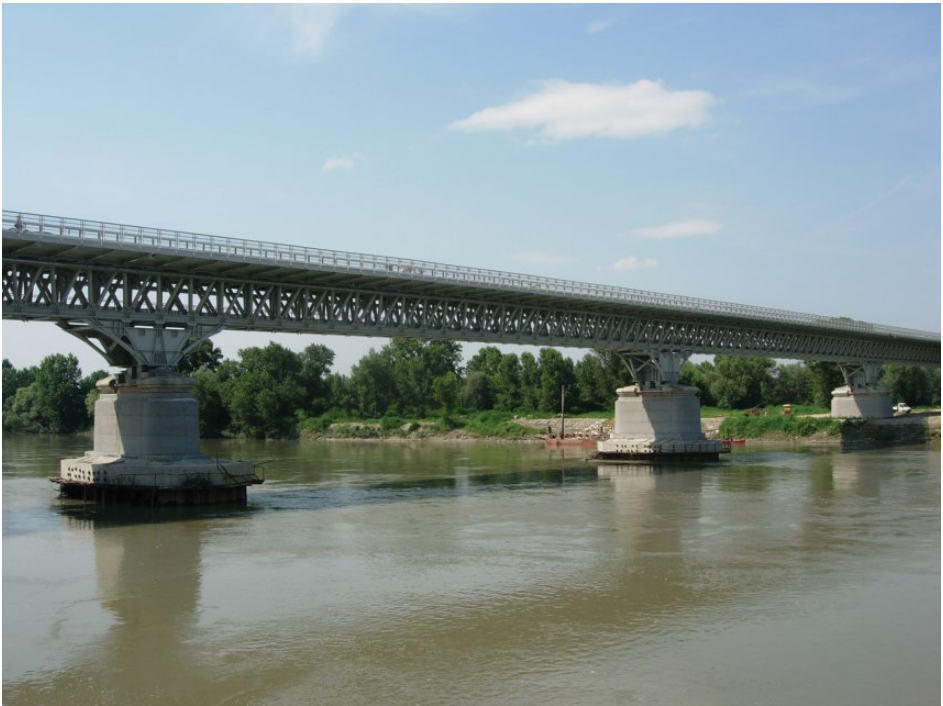
Figure 3 Using an orthotropic deck collaborating with the spatial steel structure beneath allowed a great reduction of the loads acting on the historical piers. © MCA Engineering.
